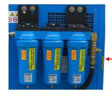
On/Off Flow Valve Handle in On Position
