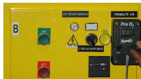
Permeate Oxygen Analyzer
