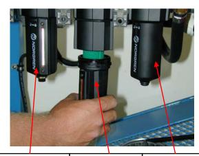
B74G Filter with Auto-Drain Float & Liquid Level Indicator F74H Filters with Auto-Drain Float & Liquid Level/ Service Indicators F74V Filter with Manual Drain – Should not Contain Moisture
