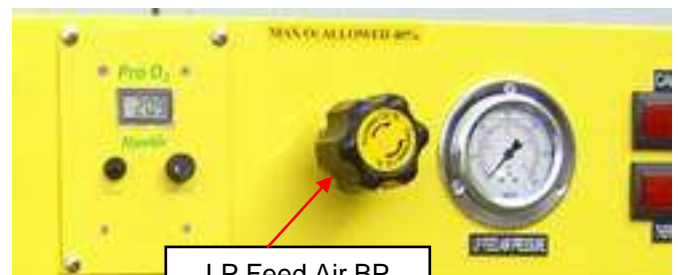
LP Feed Air BP Regulator Adjustment Knob
