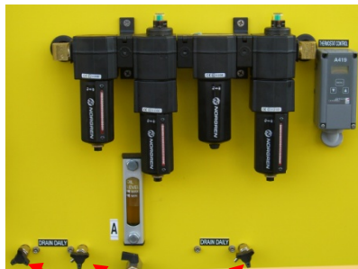
Manual Condensate Drain Valves
